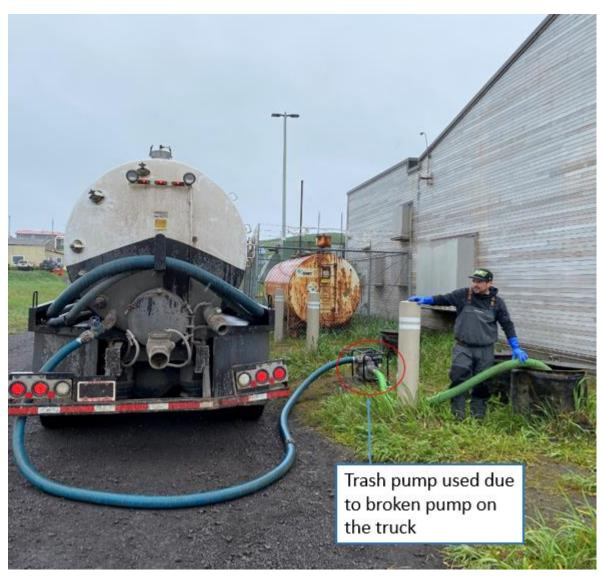
Photo 2: Trash pump used for septic pumping.
